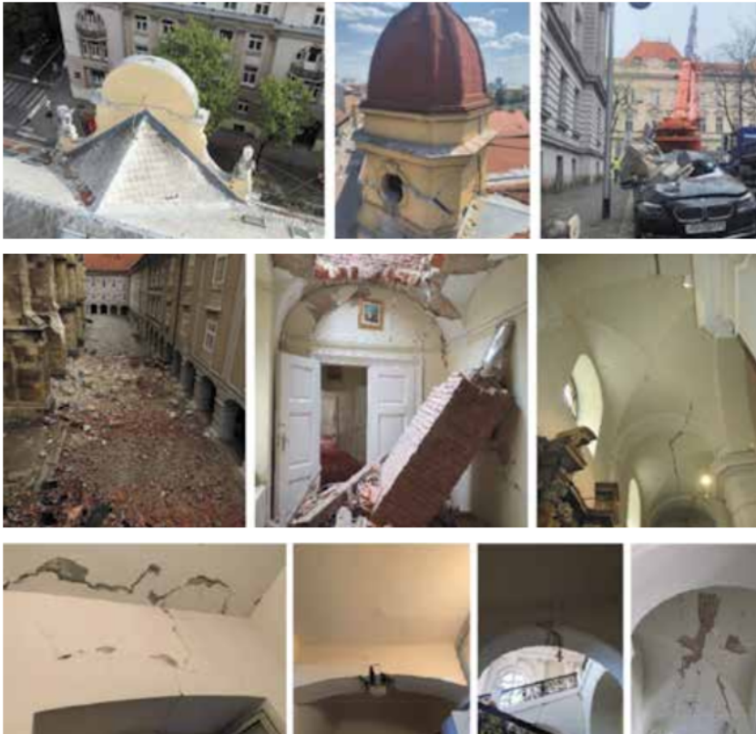
Figure 7 Consequences of the 2020 earthquake in Zagreb (Croatian Centre for Earthquake Engineering, 2024)
